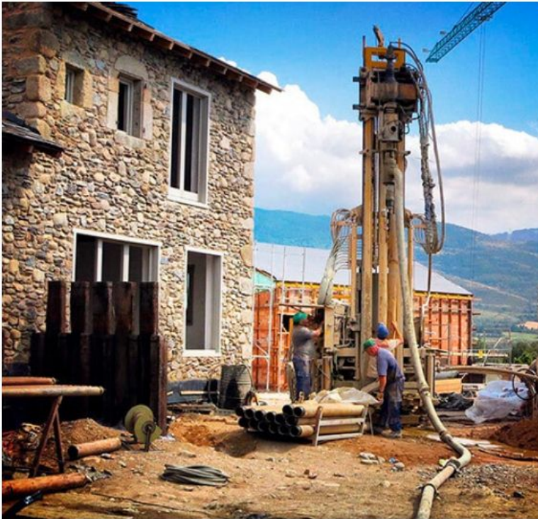
Drilling works for a vertical borehole
